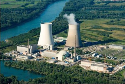
The Philippsburg nuclear power plant (Photo credit: EnBW)
