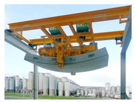
On the job: the heavy precast elements are lifted by way of air vacuums
