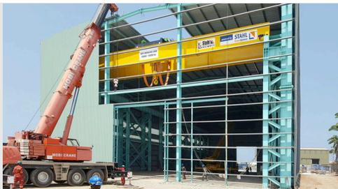
An intercontinental project: the crane system from Stahl Cranes & Hoists from South Africa was erected in General Electric's new plant in Ghana with the technology of STAHL CraneSystems from Künzelsau.
