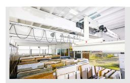
Self-supporting structure: the new crane runway protrudes more than 3 metres into the wider part of the hall. This area can be served by both cranes.
