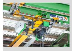
On the left: five light barriers for contactfree signal transmission between the crane bridges, top centre the chain hoist for the interlock mechanism, on the right the conductor lines for travel and logic signals.
