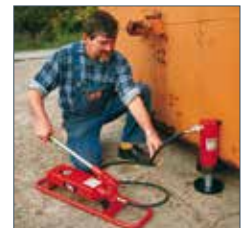
Lifting of a container by use of an hydraulic cylinder YS-23/160, lifting claw AYS-23 and piston plate AYS-232 powered by a two-stage hand pump HPS-2/2 with base frame.
