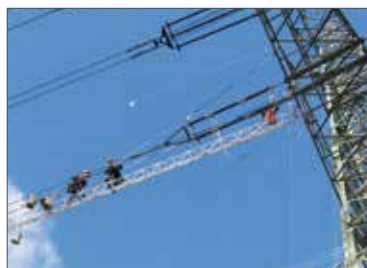
Overhead line construction
