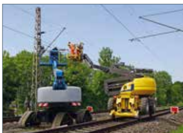
Construction of contact lines
