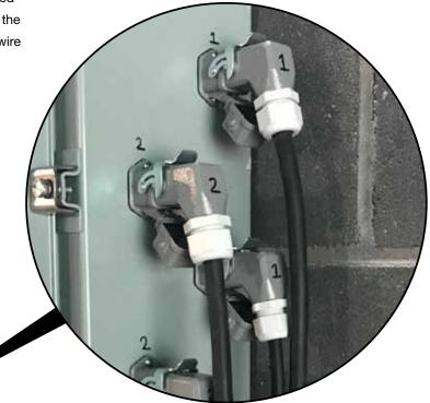
Actuator motors, limit switches, and encoders designed with quick disconnects at the controls enclosure to be quickly removed and installed to accommodate scheduled maintenance needs.
