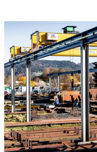
To cope with the increase in the volume and weight of material handled, the crane system in the storage yard of Stahlbau Schauenberg GmbH in Kirchzarten in southern Baden, Germany, was modernised with two double girder overhead travelling cranes with a span of 20 metres and a lifting capacity of 10 tons each.
