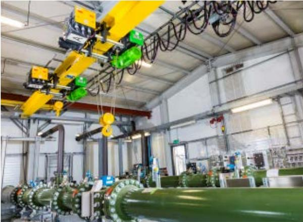
1 The explosion-protected tandem crane with two SH wire rope hoists and radio remote control is used in the construction of a compressor station for a natural gas pipeline. Both SH 40 Ex wire rope hoists are designed for safe working loads of 3,200 kg and meet the ATEX directives as regards design and safety.
