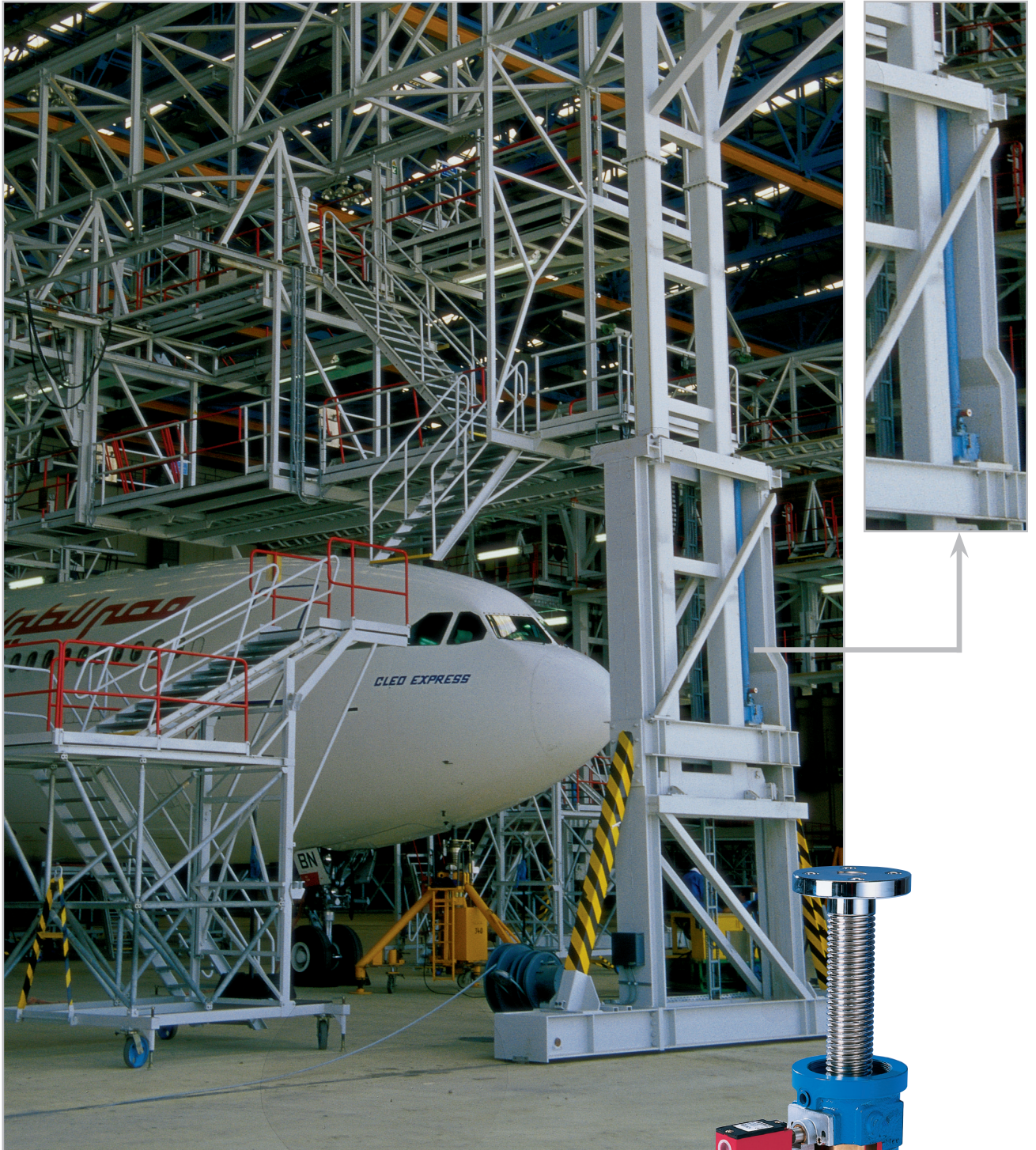
Pict.: Egypt-Air Works photo: MERO-Airporttechnik
